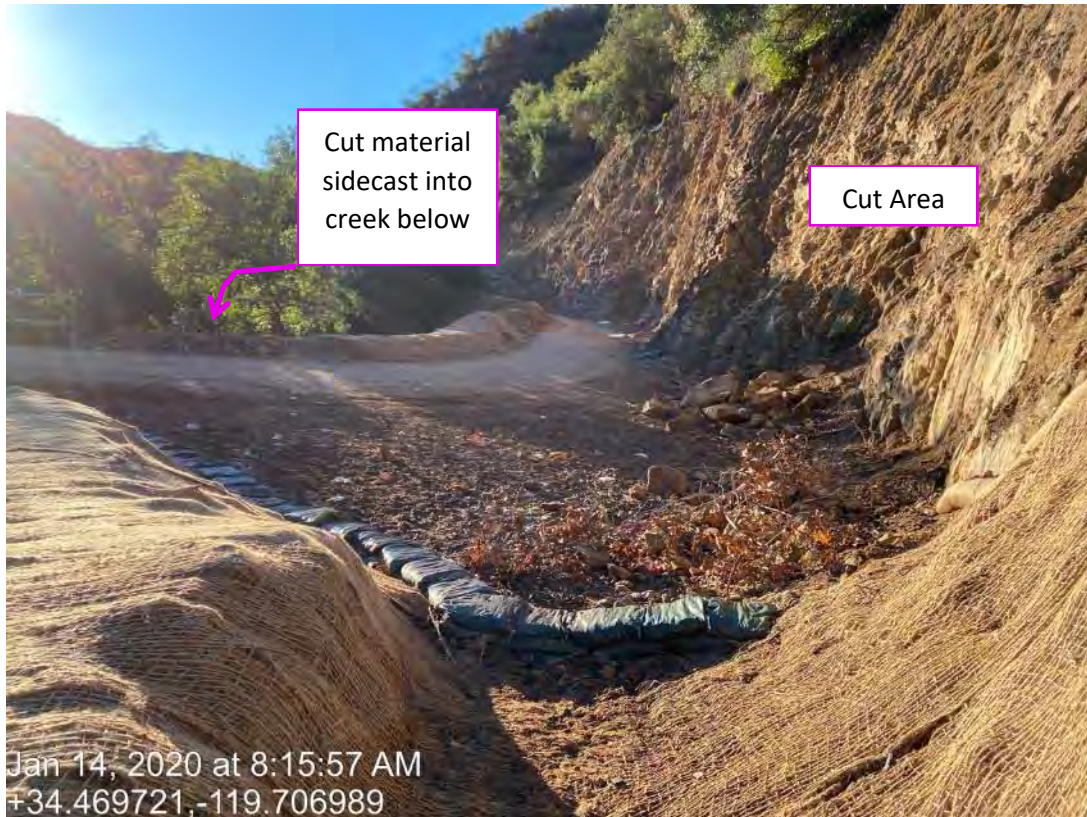
Photo 2: Cut face near bridge, looking southeast.
