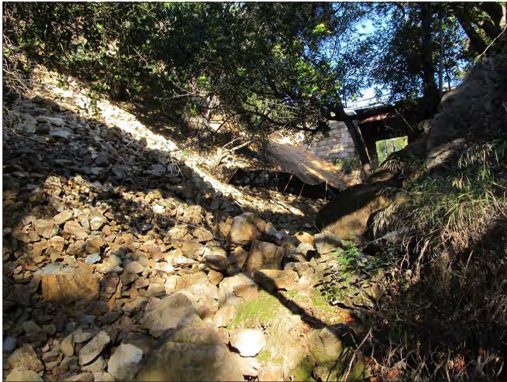
Photo 2. Looking upstream at Creek Site 2 in Mission Creek.
