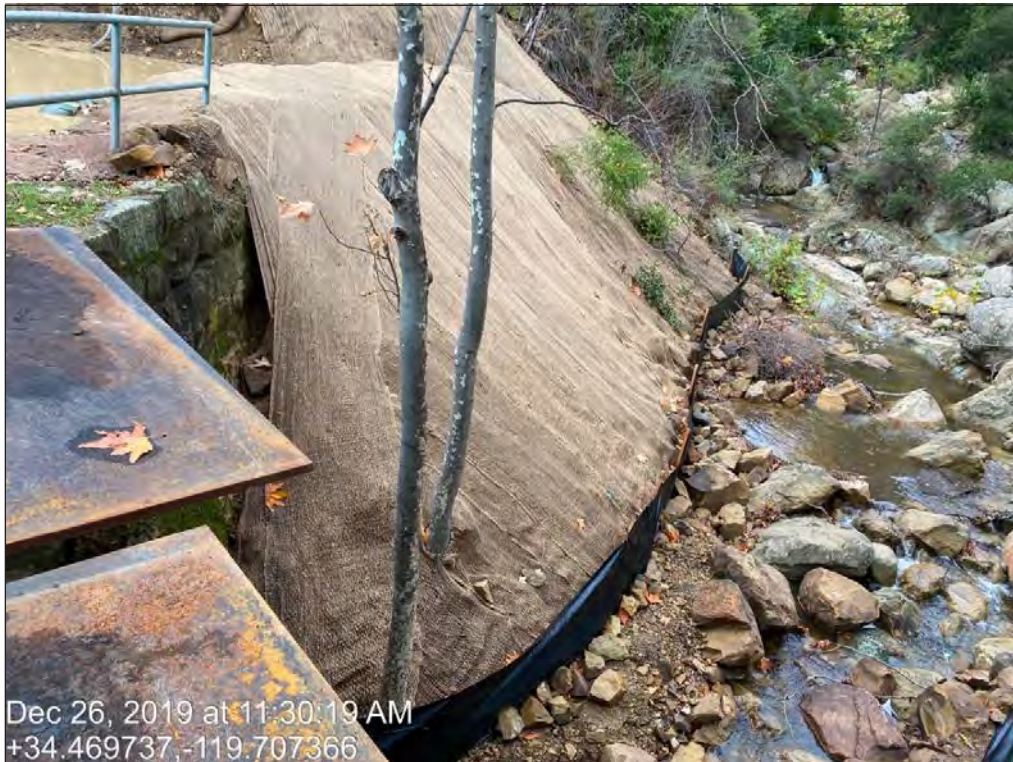
Photo 10. Erosion control matting and silt fence at Creek Site 1.
