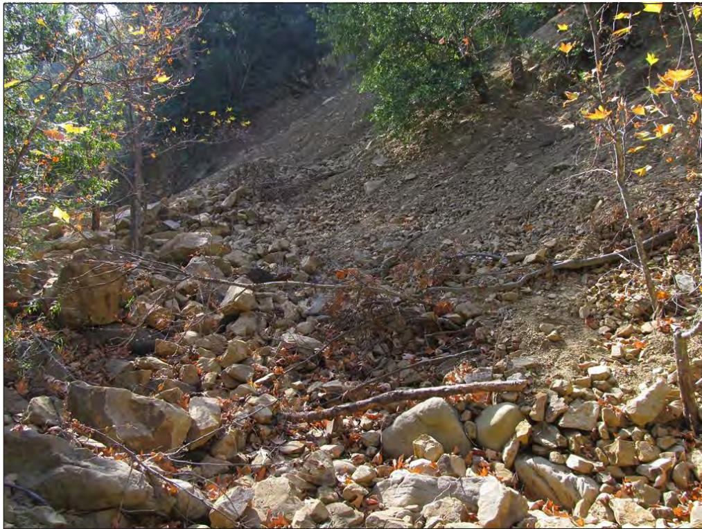
Photo 4. Looking downstream in Mission Creek at Creek Site 3.
