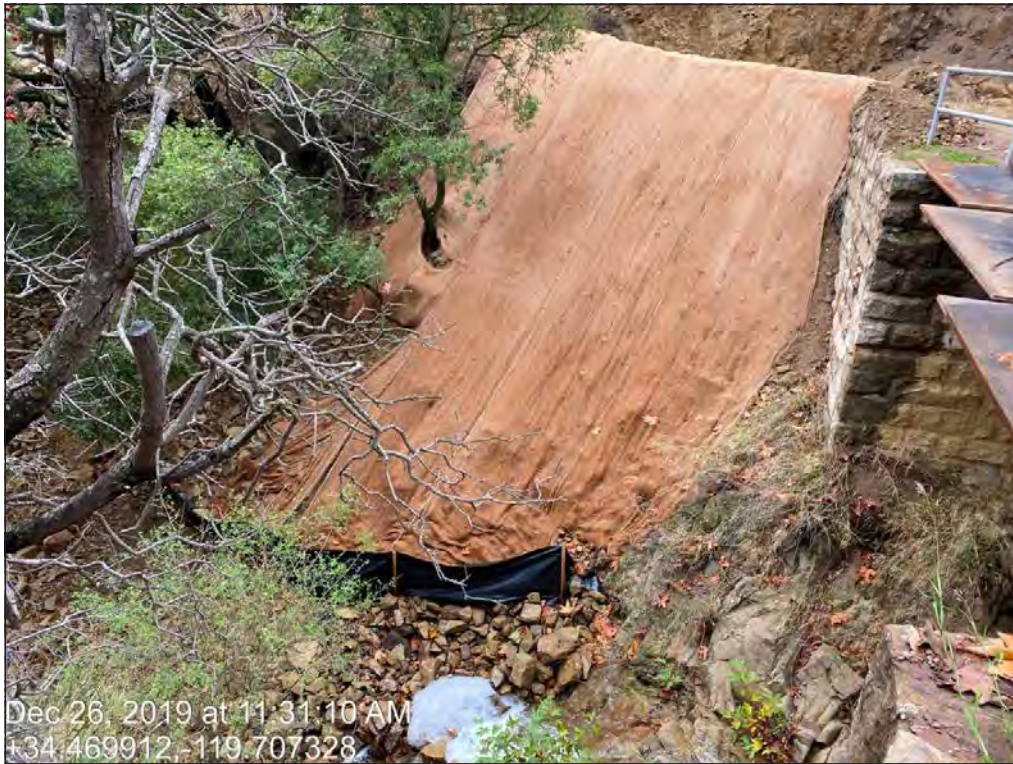
Photo 9. Erosion control matting and silt fence at Creek Site 2.
