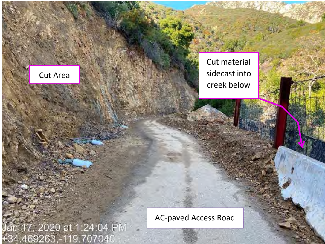
Photo 1: Cut face, AC-paved road, looking northwest.
