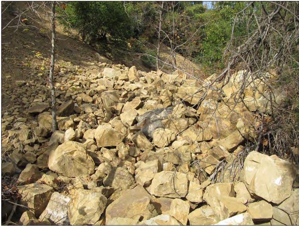
Photo 1. Example of sidecast in Mission Creek.
