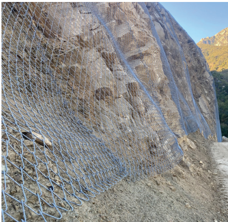
Close-up of the fencing on the rock wall.
