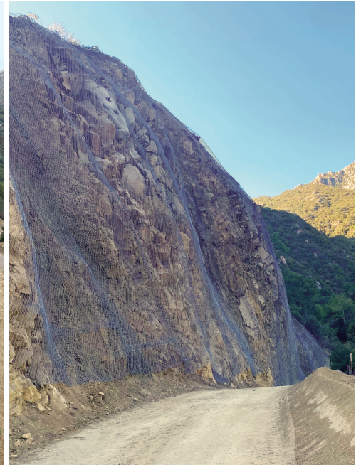
Before and After: The rock wall by the bridge before and after Edison scraped the face of the canyon wall. Edison put up wire netting to prevent future rockfall.
