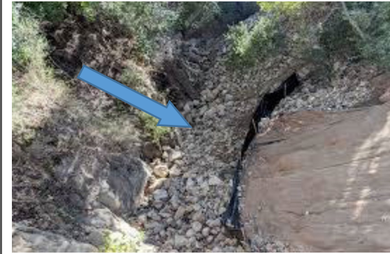
Soil and rock was discharged directly into Mission Creek
